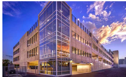
Four-level, 326-space, CIP PT parking structure. This garage was designed for future expansion and included glass-enclosed stair towers for optimal passive security. The parking facility provides crucial additional parking for the VA Sierra Nevada, Reno, NV campus.
