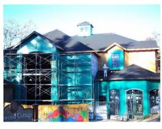
Construction is progressing with Boone Construction Company. Several items that are being added at this point in construction are: stone on the lower level of the parking structure and on the back (west side) of the structure, fluid applied membrane air barrier/vapor permeable (green material) to the exterior sheathing, and the exterior
