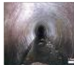
Clean sewer line
