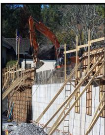
The parking facility project, off Wallingford Street is underway with retaining walls poured and pier footings excavated. This project is being funded through the TDA’s occupancy tax proceeds as well as Parking Fund in-lieu fee payments. When completed, the parking facility will provide 69 additional spaces in the American Legion area. The project is scheduled for completion in April 2009 and is currently slightly ahead of schedule.
