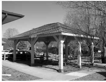
Memorial Park Picnic Shelter
