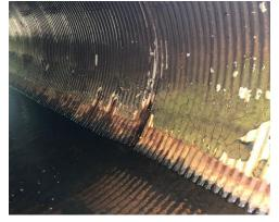
We have considered several possible options for addressing this issue, from pipe rehab to total replacement. Pipe rehabilitation can come in several forms, cement lining – centrifugally applied, slip lining with a smaller high density polyethylene pipe, or plate installation. Each method has its advantages and provides less disruption to the roadway. Full replacement would require excavation of the roadway (eliminating access for some period) and handling of the pipes that
