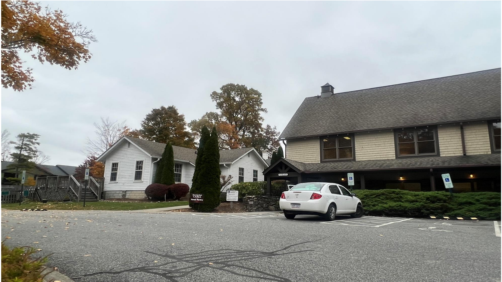
Rumple Memorial Presbyterian Church Blowing Rock, NC
