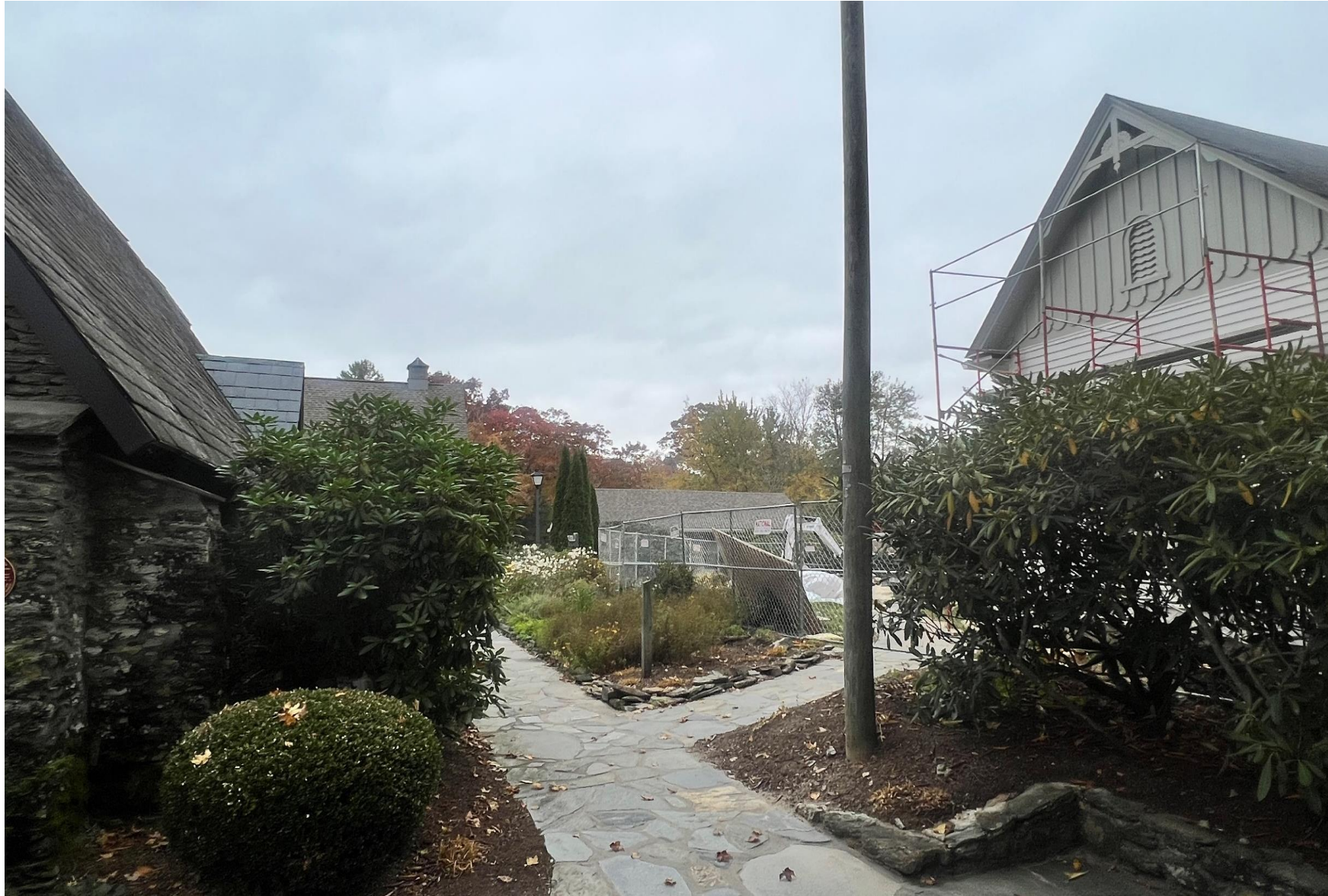
Rumple Memorial Presbyterian Church Blowing Rock, NC
