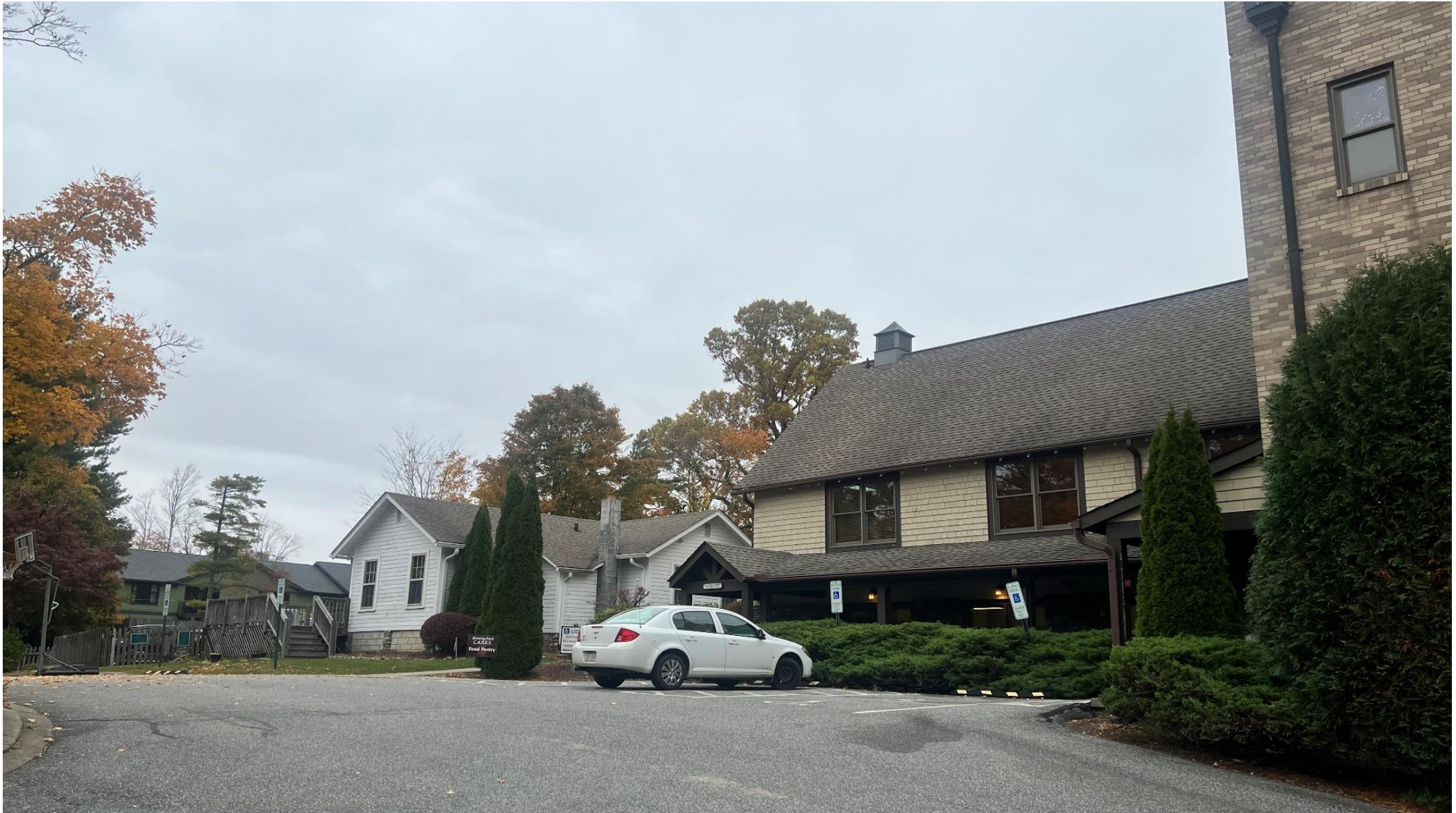
Rumple Memorial Presbyterian Church Blowing Rock, NC
