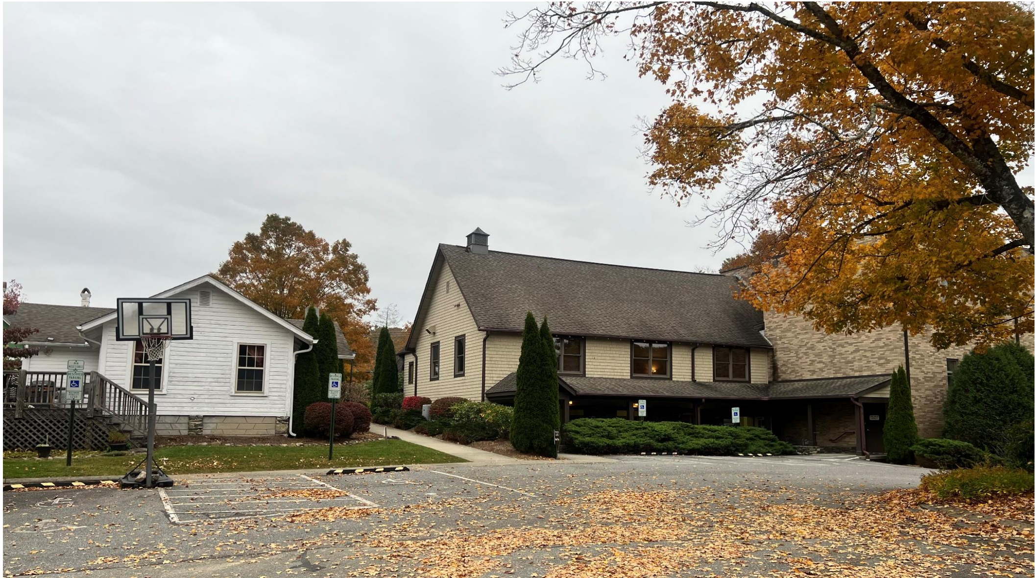
Rumple Memorial Presbyterian Church Blowing Rock, NC
