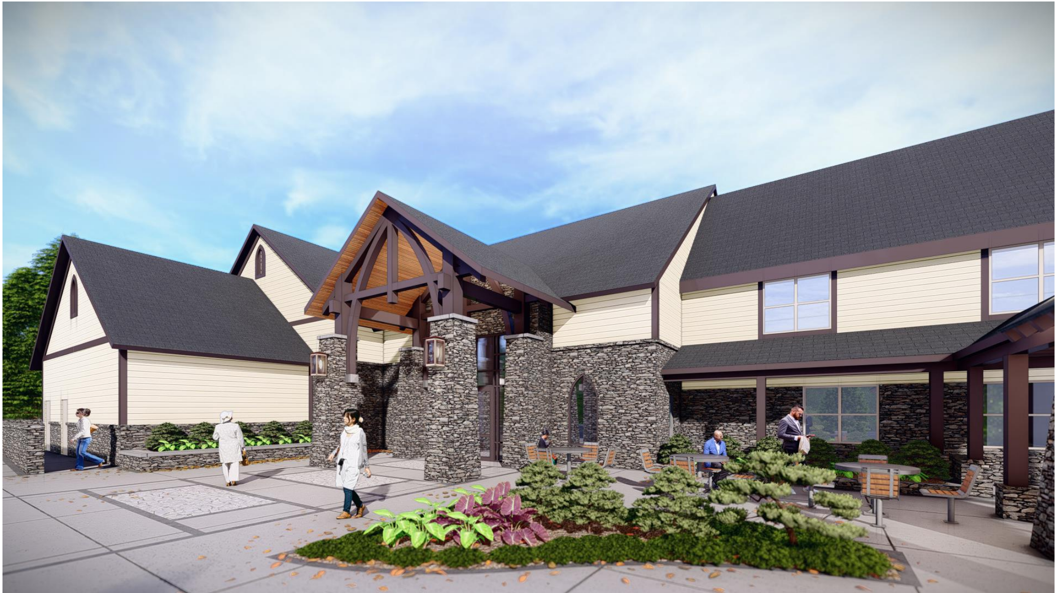
Rumple Memorial Presbyterian Church Blowing Rock, NC
