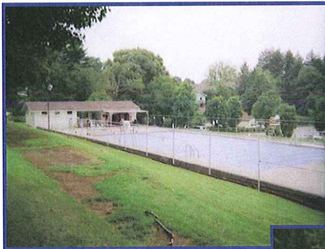
Exterior Facilities Swimming Pool Kiddie Pool Picnic Area Pump House Parking
