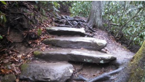
Example 4 – Failed stone stairs
