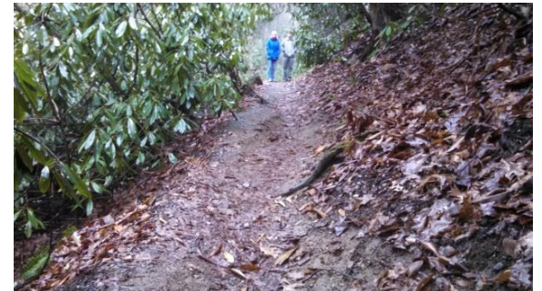
Example 6 – Drainage problems
