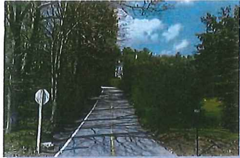
Morningside Drive Facing North Near US 221
